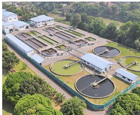
Figure 8.1 Wastewater Treatment Plant in Kandy Municipal Site
